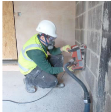
Figure 5: PPE and Controls; wall chasing using on-tool extraction [7]
