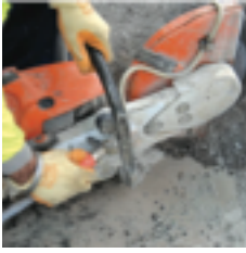
Figure 8: Controls; water suppression on a cut-off saw [7]
