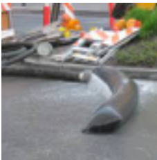
Figure 13: Environmental controls; filter socks
