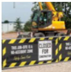
Figure 17: Environmental controls; site fencing filter wrap
