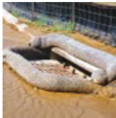
Figure 14: Environmental controls; filter socks
